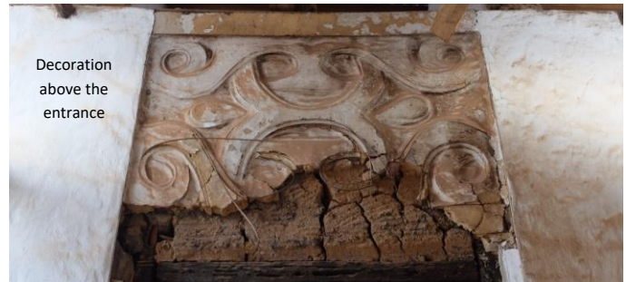
Partially restored roof, inappropriate cement plinth, poor drainage on the southern side badly restored decorations and broken decoration above the entrance.
