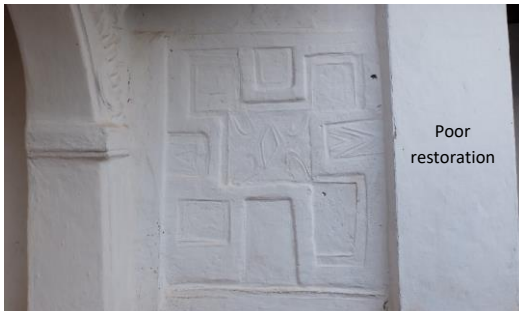
Partially restored roof, inappropriate cement plinth, poor drainage on the southern side badly restored decorations and broken decoration above the entrance.
