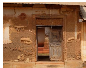
Very fragile roof, eroded drainage slopes, eroded wall bases and damaged decorations
