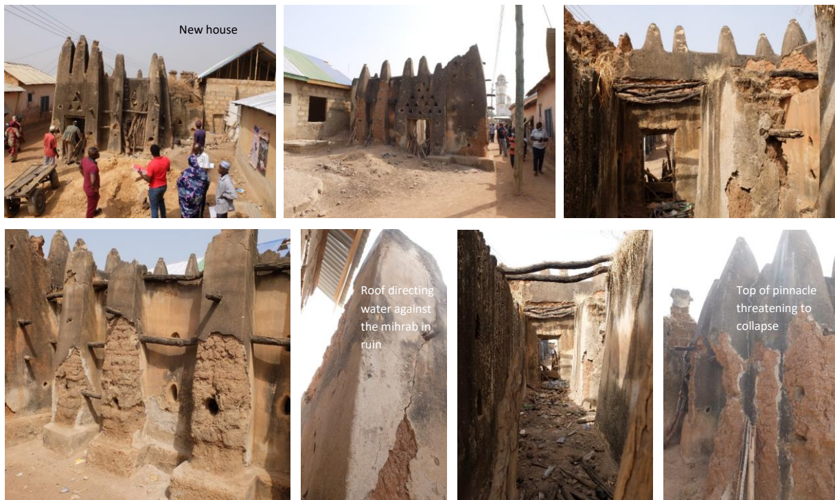
Remains of Dondoli mosque. The walls are almost intact but the roof is gone
